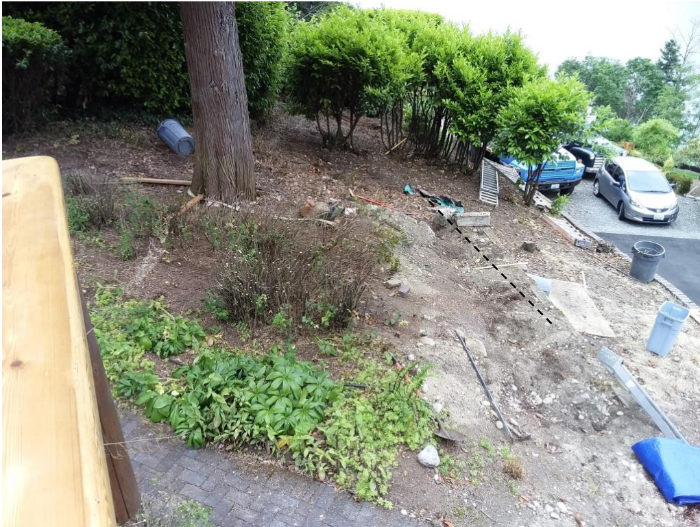
Figure 10. Photo showing the location of the retaining wall on the west side of the #13 cedar (black dashed line).
